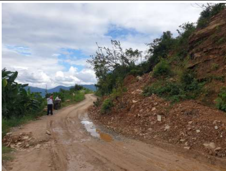
Photo 12: Landslide area at Chainage 2+640 to 2+700 of Section I
